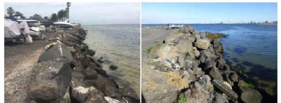
FIGURE 7-2 WESTERN SEAWALL: SEAWARD OF HARDSTAND AREA (LEFT) AND AT THE MARINE ENTRANCE (RIGHT)
