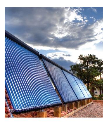
Solar thermal can describe any system in which solar radiation is used to directly heat a medium that can retain and use the heat such as water, air, or solid wall.
